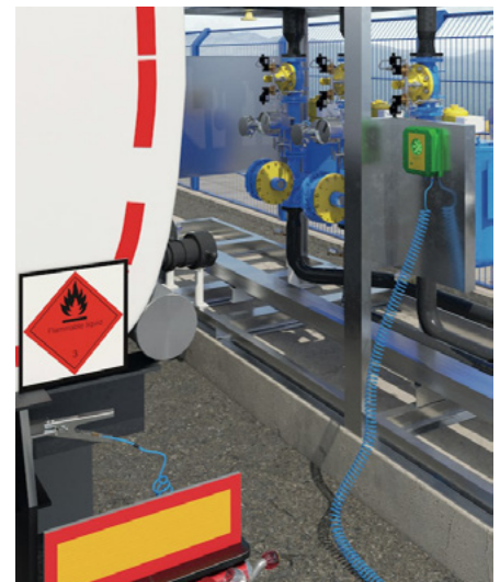
Fig. 4: Grounding monitoring of a truck by means of FARADO II
